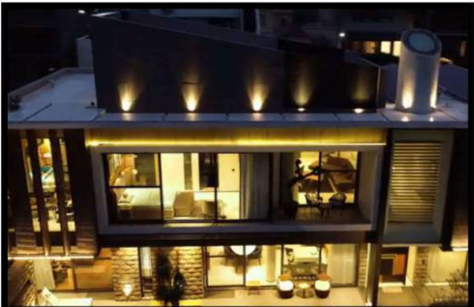
Project : Bungalow at Chandigarh by Architect Harpreet Singh
